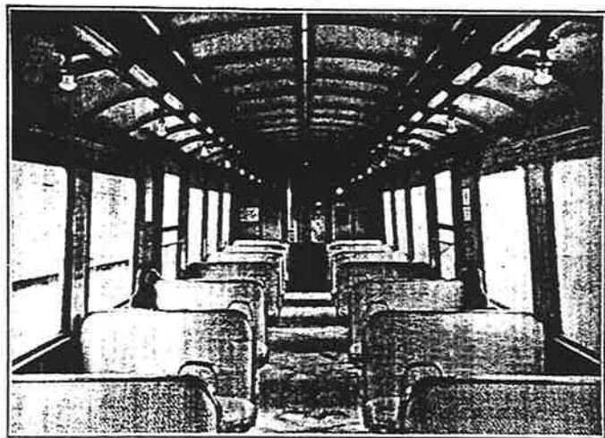
A London Underground Railway Carriage with "Tantalum" Lamps installed.
